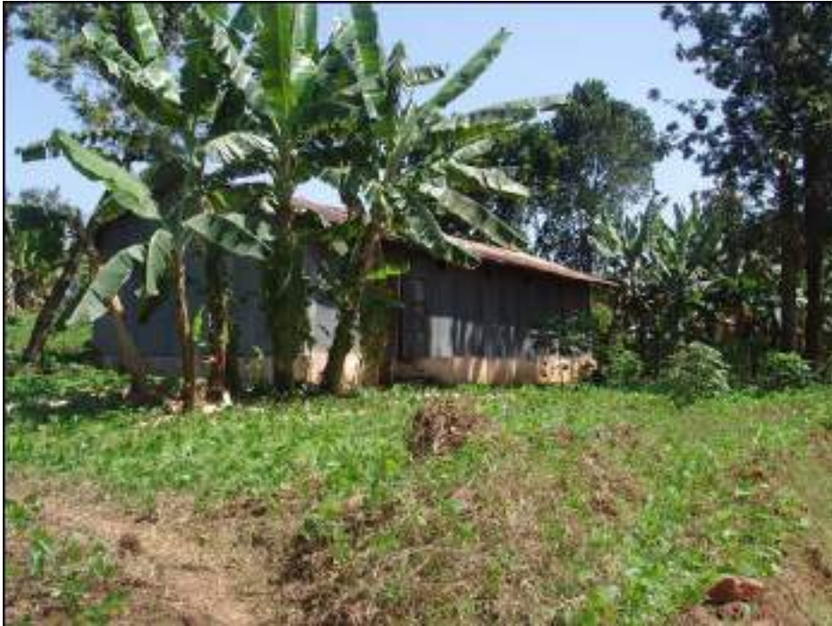
Figure 9: Armory building made of iron sheets used by Tanzanian soldiers still stands intact at Minziro village.
